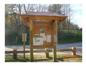
This heavily constructed kiosk includes a railroad station-type roof of split cedar shakes and pressure treated lumber construction. The display board cover is plexiglass and hinged and lockable. This style is used throughout the Farmington Canal Heritage Trail and River Trail system.
