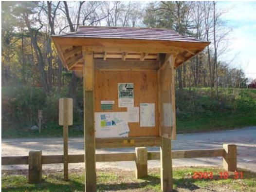
This heavily constructed kiosk includes a railroad station-type roof of split cedar shakes and pressure treated lumber construction. The display board cover is plexiglass and hinged and lockable. This style is used throughout the Farmington Canal Heritage Trail and River Trail system.
